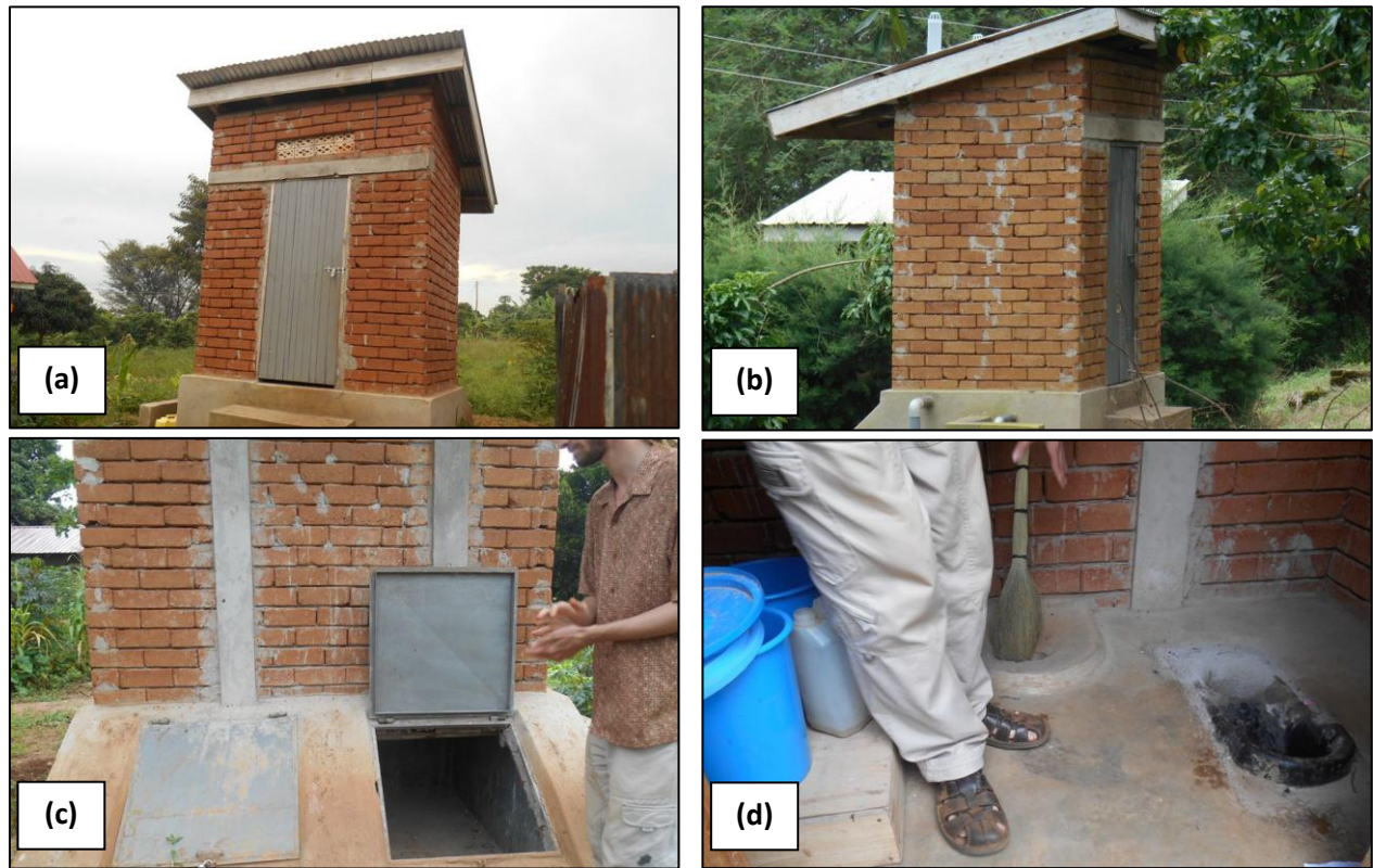
Figure 4: Demonstration UDDTs installed in primary schools in Kalisizo, Uganda (all photographs taken by Debra Trimmer). (a) External front view; (b) external side view; (c) external rear view, showing two fecal collection vaults; (d) internal view, showing the urine diversion device
